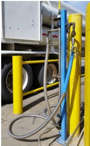
Designed specifically for the ultra hazardous applications of high pressure hydrogen gas transfer in tube trailers, facilities and cylinders. Whether you prefer metallic or Tefzel®, the LifeGuard hydrogen hose is the Safe-Choice.™ The inner hose, braid, armor casing cuffs, weld ring, and ends are all stainless steel. Each finished assembly is pneumatically tested to ensure it will withstand the application requirements.
